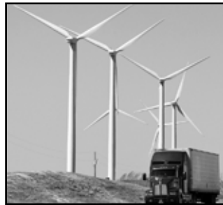
Lots of truck traffic during the drive but this wind farm in Texas was unique and added some interest to an otherwise rather boring drive
